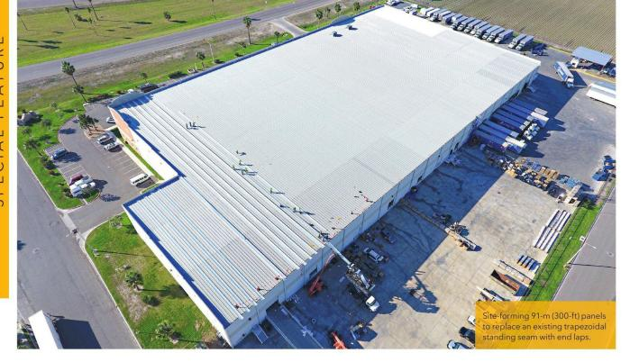
Over the last few months, contractors have seen between 2.26 and 5.44 kg/m<sup>2</sup> (5 and 12 lb/sf) of additional capacity added to the purlins in an existing building. This is a huge deal. Instead of just looking for the most economical solution to make the roof stop leaking, contractors are having discussions about fortifying the structure and adding insulation, ice and water shields, and even solar along with a new watertight roof.
